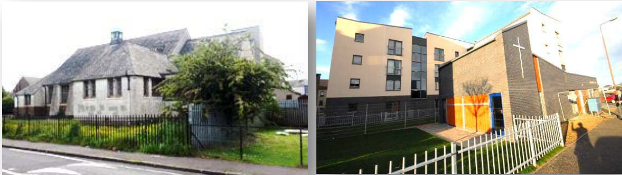
Figures 13 and 14: Granton United Church in Edinburgh. Original (left) and redeveloped (right).
