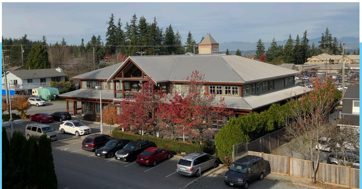
The Treehouse and its parking lot, as seen from Chorus
