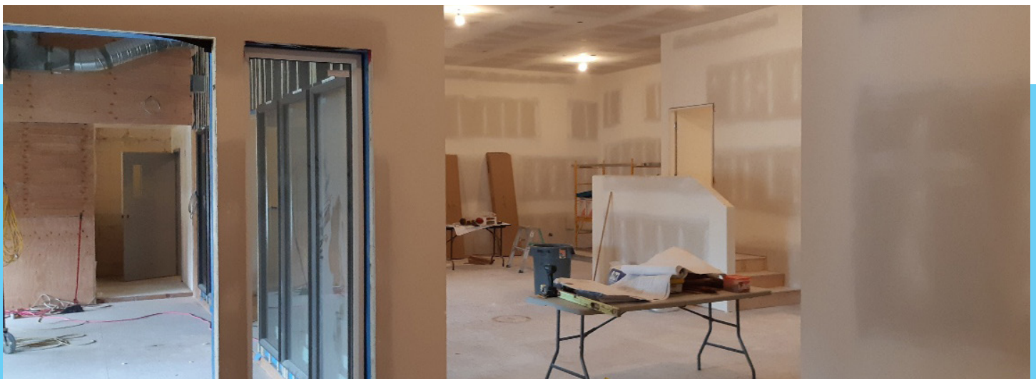
Renovations to the 4,500 sf daycare on the second floor and the 4,000 sf below it are expected to be completed in 2020. 47
