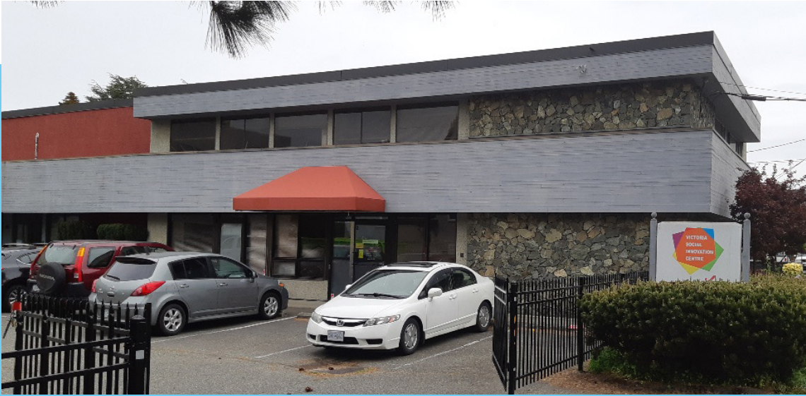
A portion of the VSIC exterior 45
